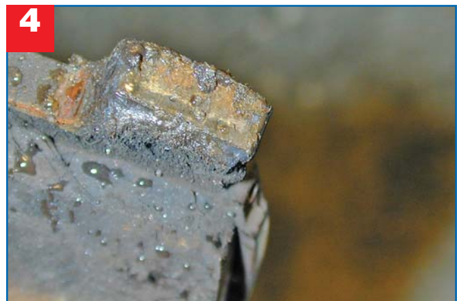
Looking at the edge of the pad shows that it has been moving and was not rusted in place.
